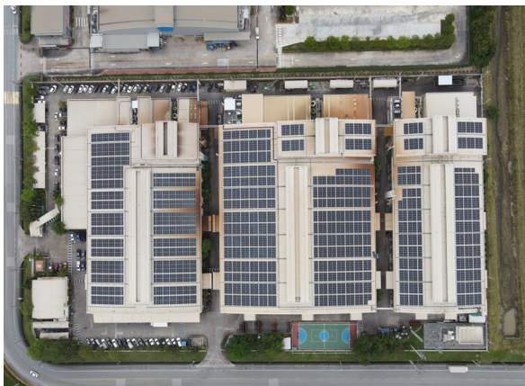
Figure 4 Picture of solar power installation of SAT-2 Plant with installed capacity of 1.5 MW
