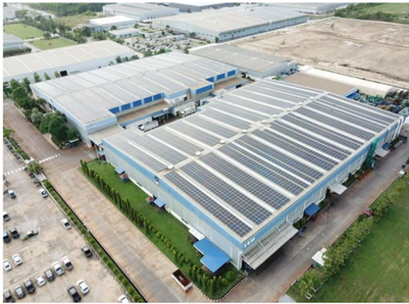
Figure 3 Picture of solar power installation of SBM Plant with an installed capacity of 1.5 MW
